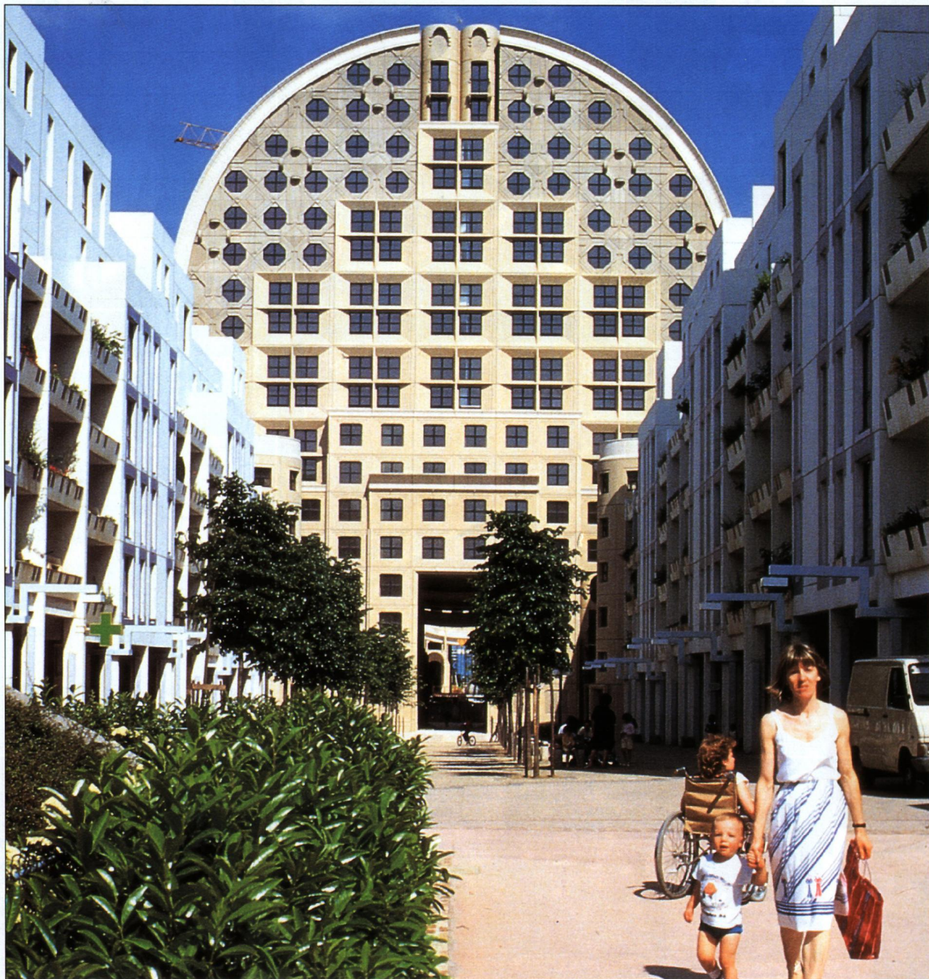
The Pablo Picasso Place in Noisy-le-Grand, near Paris, France – one of the first projects to be completely prefabricated architecturally.
